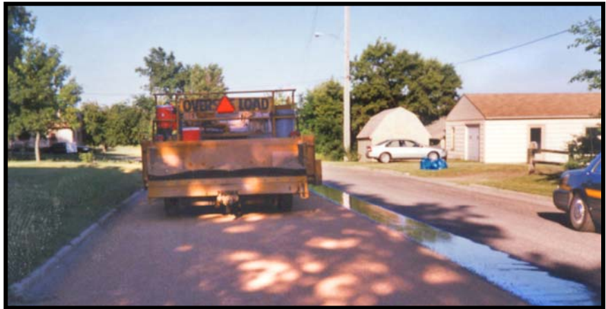
Photo 4 – Rear of the rock-chip spreading machine.
