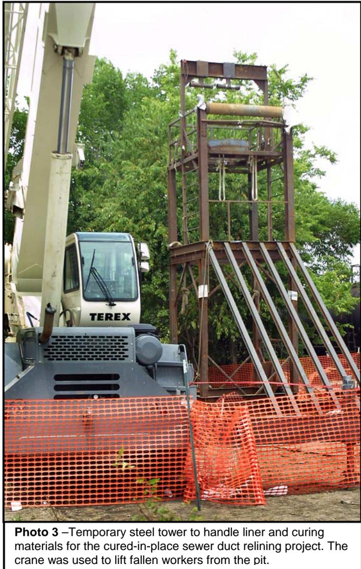
**Photo 3** –Temporary steel tower to handle liner and curing materials for the cured-in-place sewer duct relining project. The crane was used to lift fallen workers from the pit.
