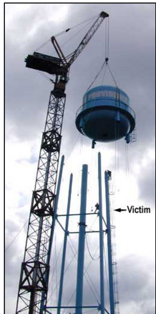
Photo 1 -- Picture of water tower taken a few minutes before the incident.
