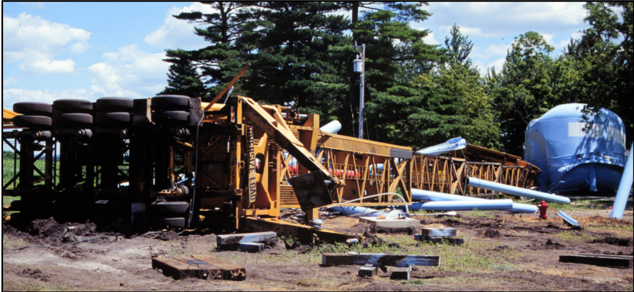
Photo 2 -- View of the crash scene taken during investigation -- photo shot from the rear of the crane trailer.
