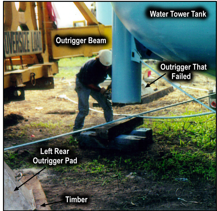
Photo 4 -- Tank worker preparing leg of the water tank.
